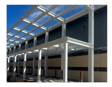
In addition to the structural steel supporting the hangar and weapons shop, this coating project also included protecting steel racks beside the structure.
