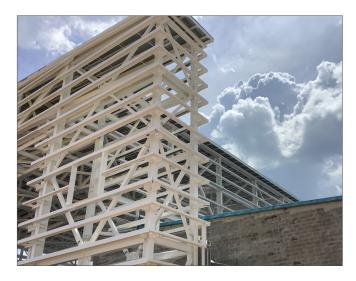
Far more of this coatings project was completed by brushing and rolling by hand than was planned. This was partly due to weather conditions including periods of strong winds. Wind contributes to the risk of foreign object debris (FOD) which must be prevented near active runways.
